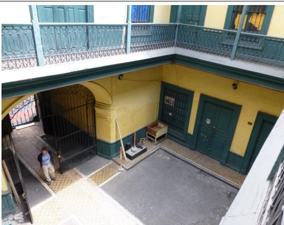
Vista del patio principal
